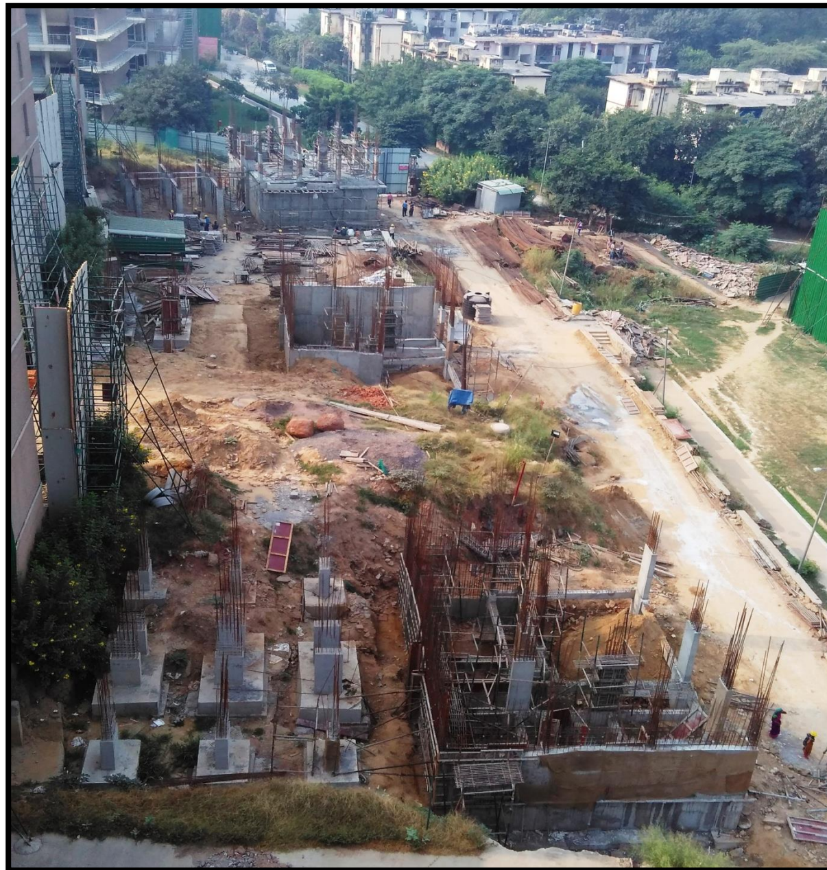
Extension Hostel Blocks G1, G2 & B1
